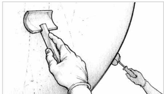
Figure 15-2 Tip off each batch, as soon as it is applied, by dragging a roller cover brush lightly over the wet surface.
